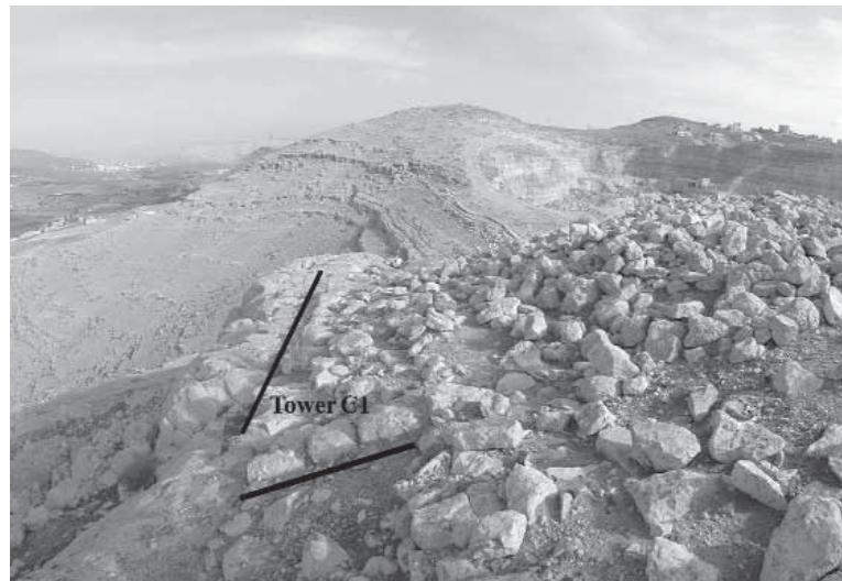
Fig. 3: The stone basement of the rectangular tower erected in the north-western corner of the site (Tower C1), from south.
